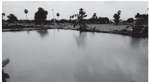
Storing the water in unlined ponds
