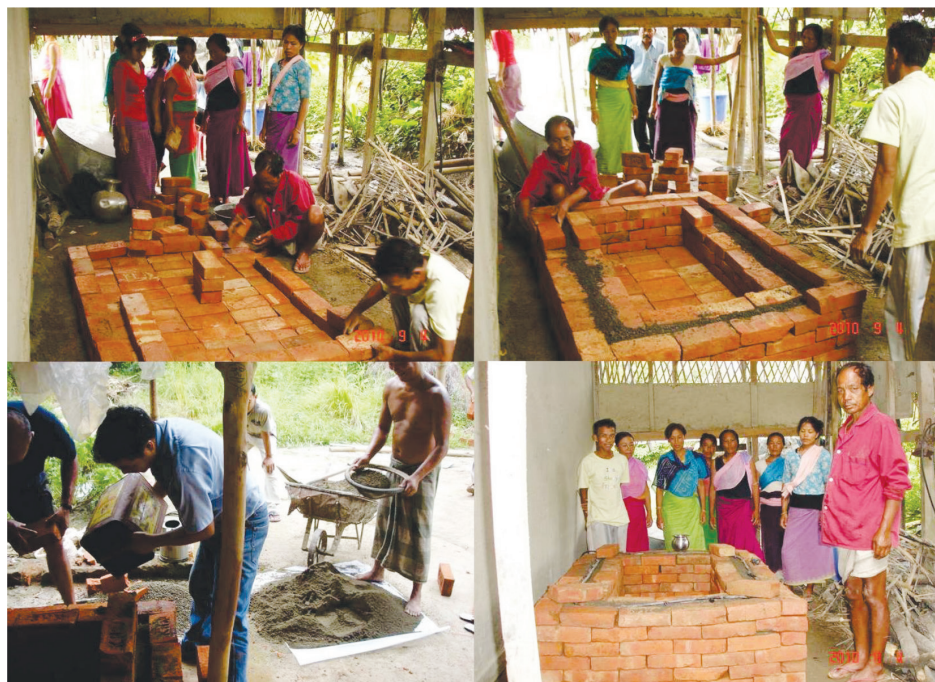
Fig. 2. Different stages for construction of zero energy cool chamber
